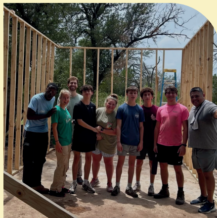
Getting walls up!
